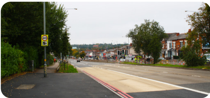
The A45 Coventry Road is a three lane dual carriageway which is a major barrier to the site
